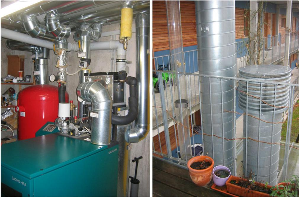
The bio-gas generator in basement, and supply and extract pipes at 'Wohnen + Arbeiten' mixed-use building in Vauban, Freiburg, 2006
